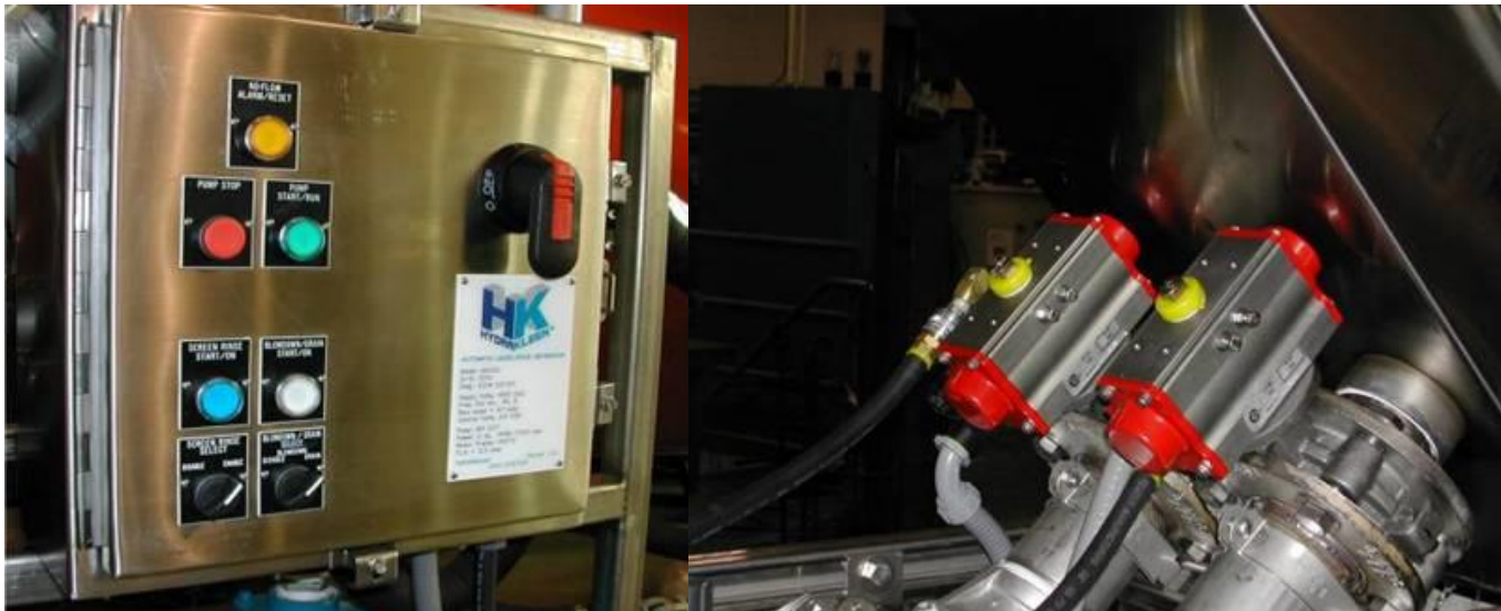
Auto Rinse Valve & Auto Drain Valve
